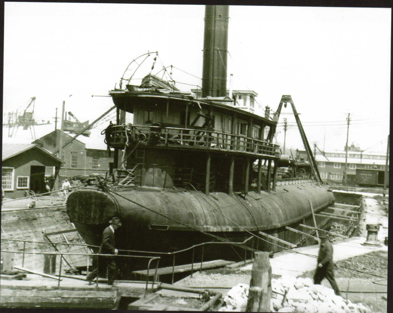
Clifton in dry dock for conversion to self-unloader.
